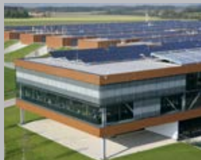
/ Fronius production and logistics site in Sattledt, Austria
